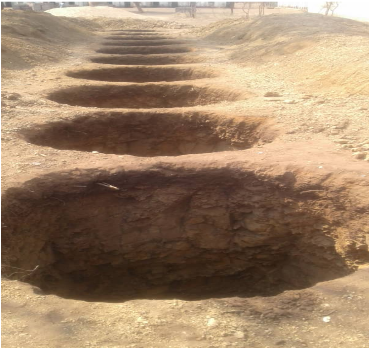
Excavation completed at Gotora primary in ward 22 Buhera
