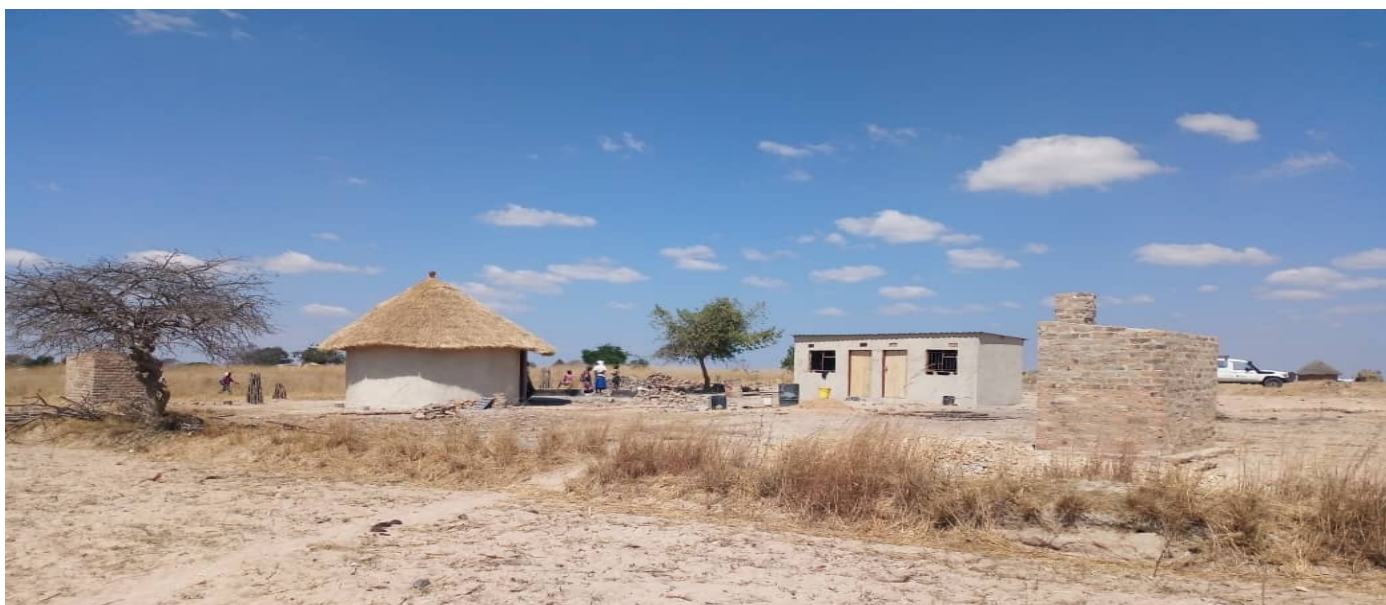
Mr and Mrs Evans Paradza Unyai's homestead completed. The model house has the full shelter package consisting of a two roomed flat house, round hut kitchen, latrine and protected deep well (pictured below).
