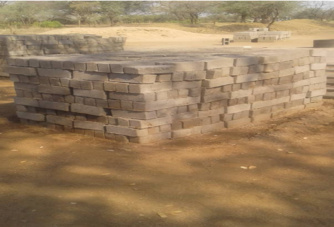
Construction material in place at Mwanyisa primary ward 24 Chipinge district
